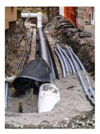
Excavating suspected pipeline leak in area where previous repair. The pipeline contained petroleum under high pressure.
